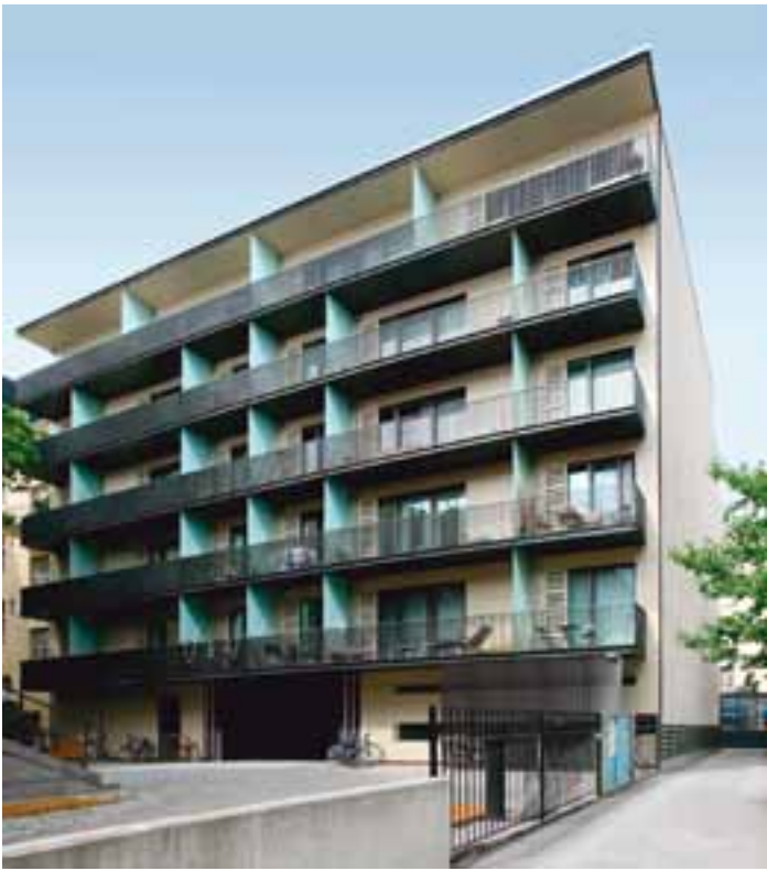
Swisspearl's light, beautiful uniform colour and form gives a modern look to the remodelled building.
