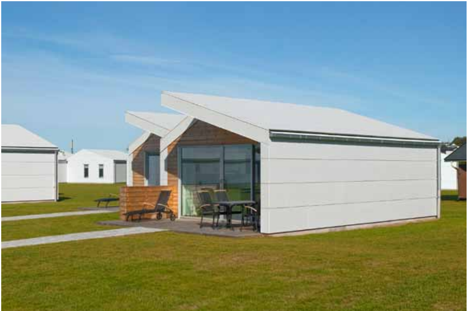
Façades and roof are merged into one single form and are covered with the same cement composite panels.
