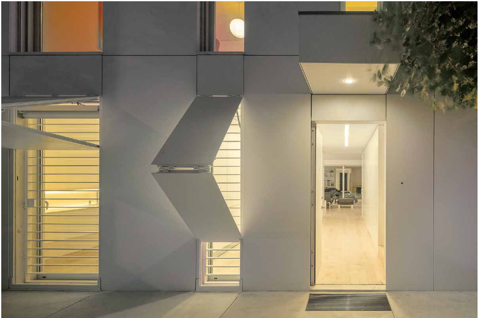
Vertical concertina shutters, enable the ground floor façade to be shut off from the street.
