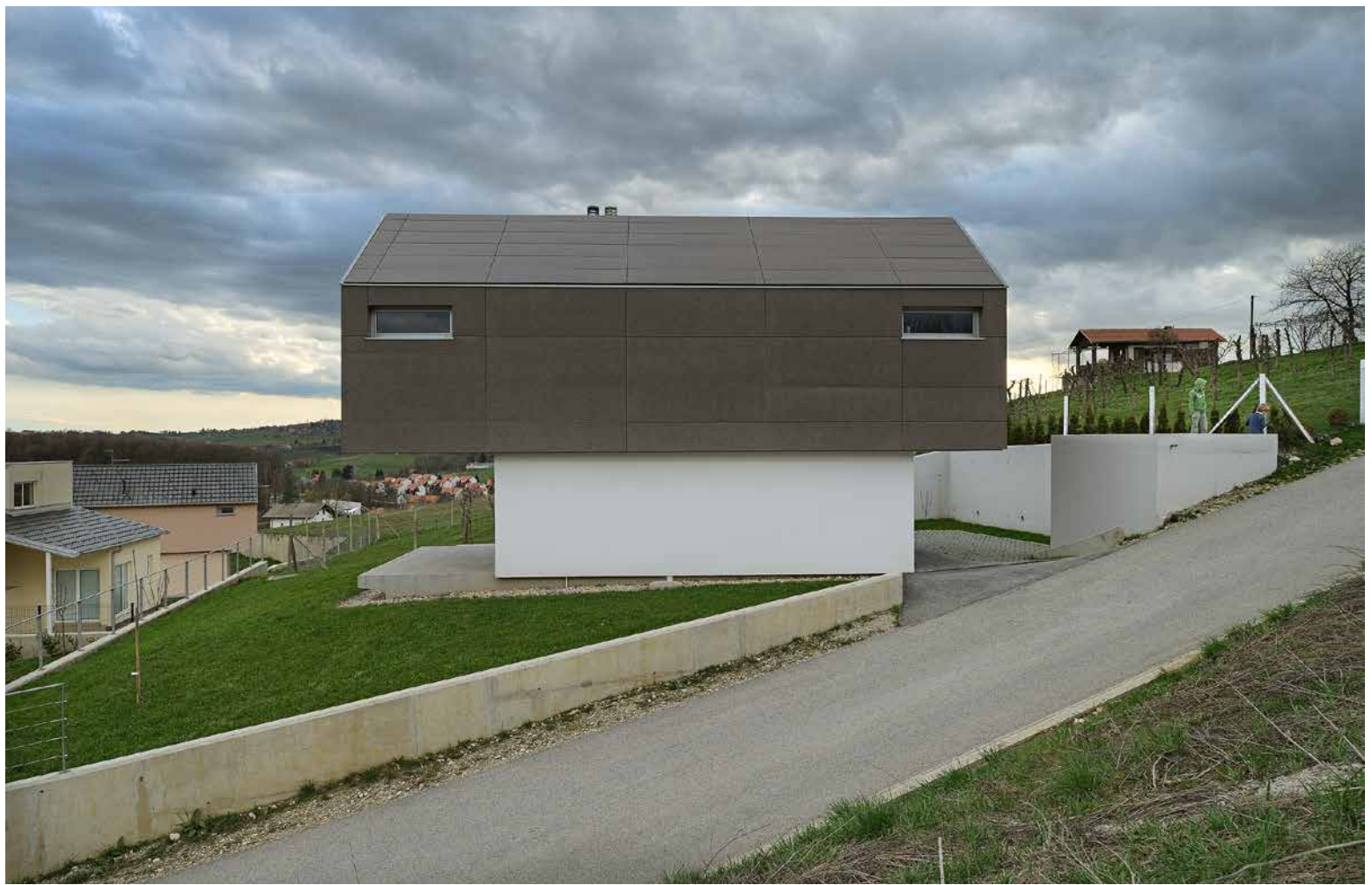
The sheltered garden terrace serves as a spatial and functional extension of the kitchen.
